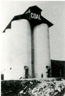
Syosset Coal Tower, not dated
